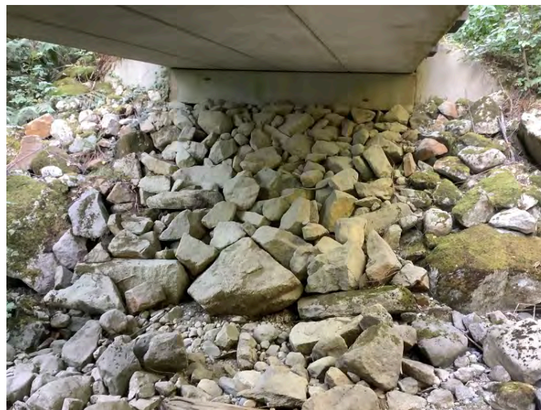
Right Bank Abutment when facing downstream
