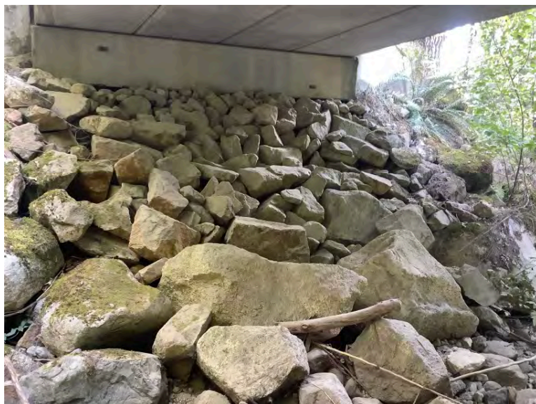
Left Bank Abutment when facing downstream
